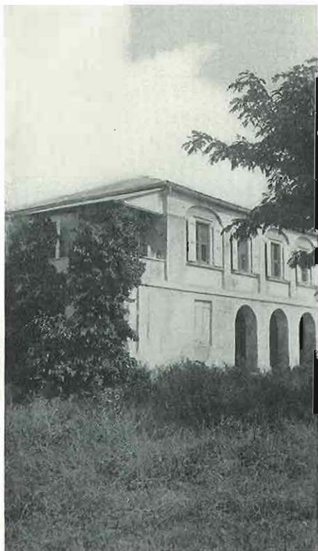
FIG. 3.—A Remodeled "Great House." This view of the owner's home on Prosperity Estate gives some idea of the old colonial "great house." It is a structure with heavy stone walls which have been given a coating of white stucco. Two stories with ceilings at least fifteen feet high were built over a full basement. The floor space includes an area of fifty by one hundred feet without allowing for the spacious porches and wide outside steps. Among the many large rooms there are bedrooms twenty-four by thirty feet, a dining room twenty-four by fifty feet and a living room twenty-four by thirty-six feet.
